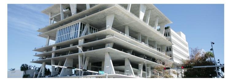
**Picture 1**. A multi-storey car park in Miami Beach also plays host to parties, yoga classes and weddings. The concrete building with floor slabs supported on wedge-shaped columns was completed in 2010 to offer naturally lit parking levels that can also be used for other activities above a row of shops and restaurants.
